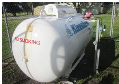
Correct installation showing first stage regulator
