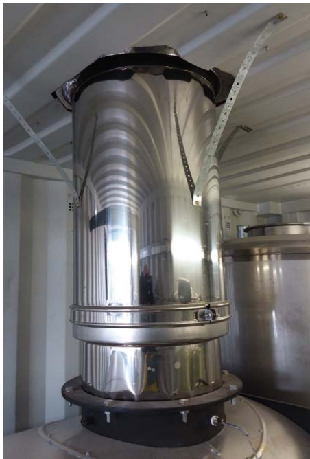
Independent supports and bolted sleeve so that appliance can be removed without disturbing the roof seal
