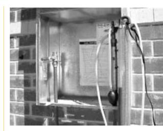
Turning the gas supply on and then off again in not an approved method of testing. In the case of LP Gas installations, this method of testing will not indicate a small leak. The pressure in (Continued over page)
