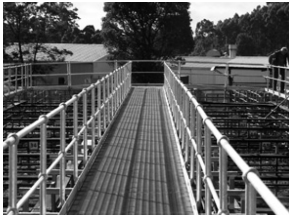
7. Animal sales yard, showing correct use of handrails and edge protection.
