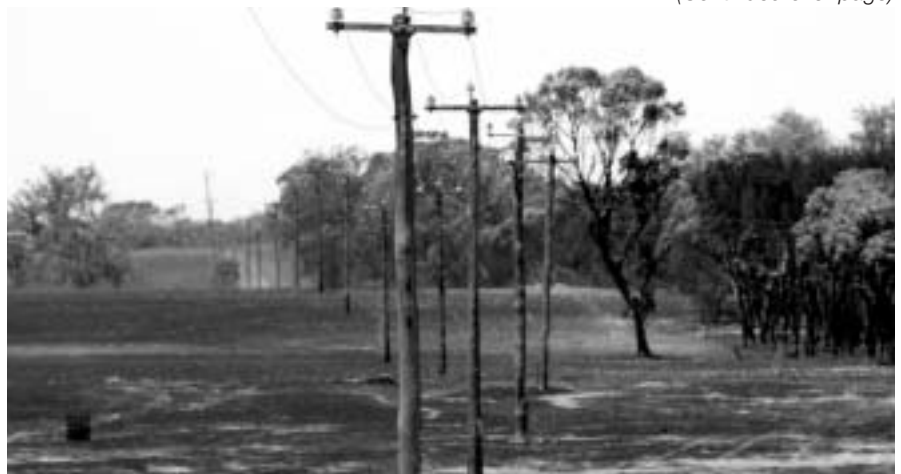
Fire damage to the Tenterden power line
