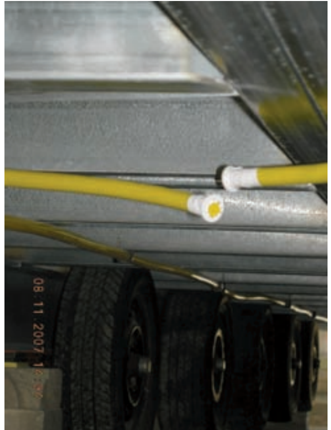
Composite pipe ready to be connected
