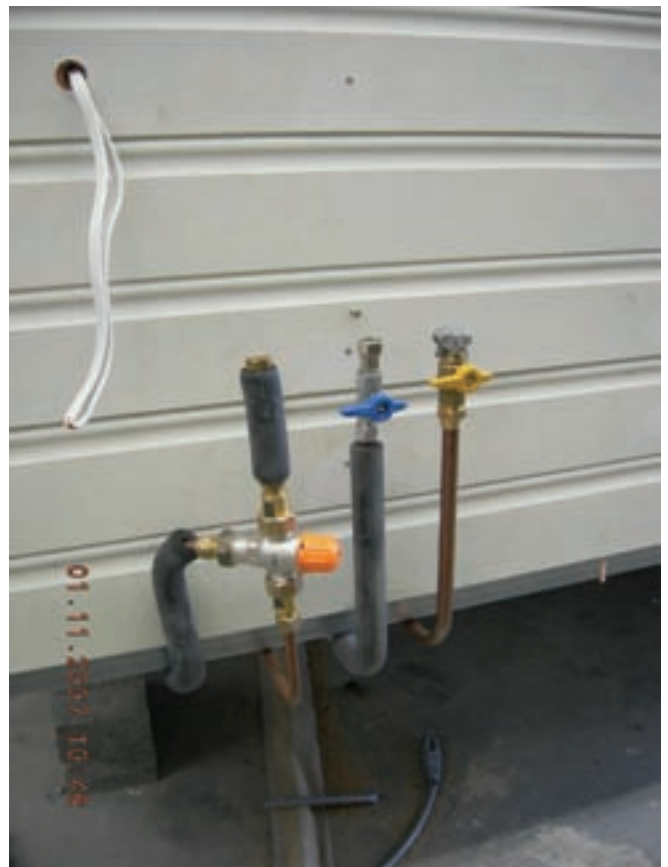
Water and gas piping ready to be connected
