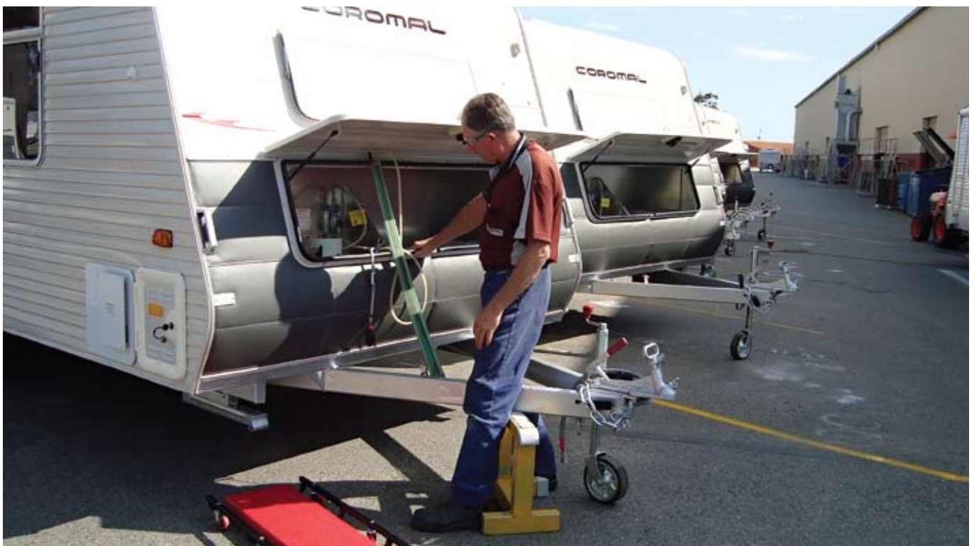
Terry Dods pressure testing the gas installation
