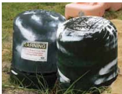
Photograph showing a poorly painted working end pillar that has the warning label peeling off.
