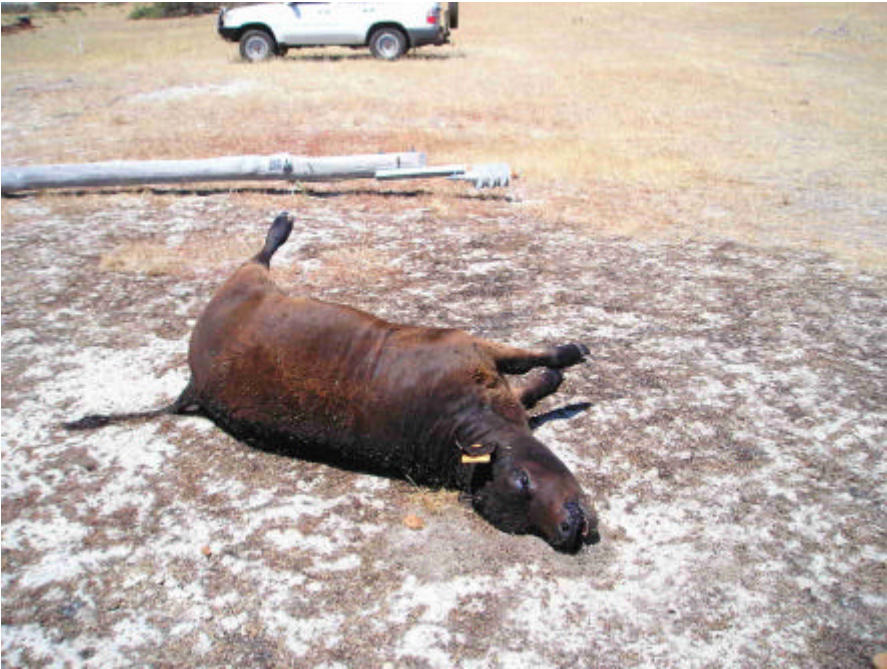
Photograph of Fire Scene with Original Wood Pole (D577/4 east) and Dead Calf
