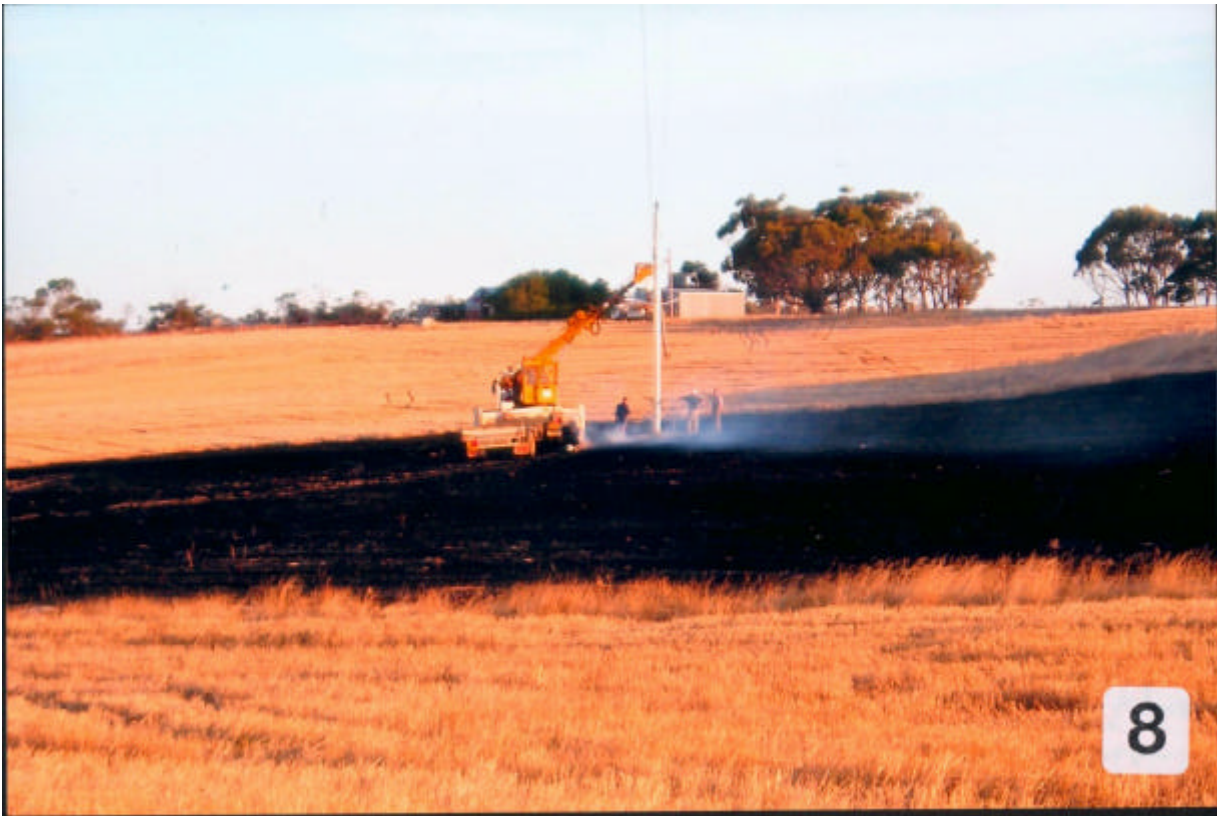
Photograph Showing the New Replacement Steel Pole (D318/35/10/8)
