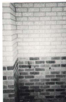
The water heater was initially connected in this recess
