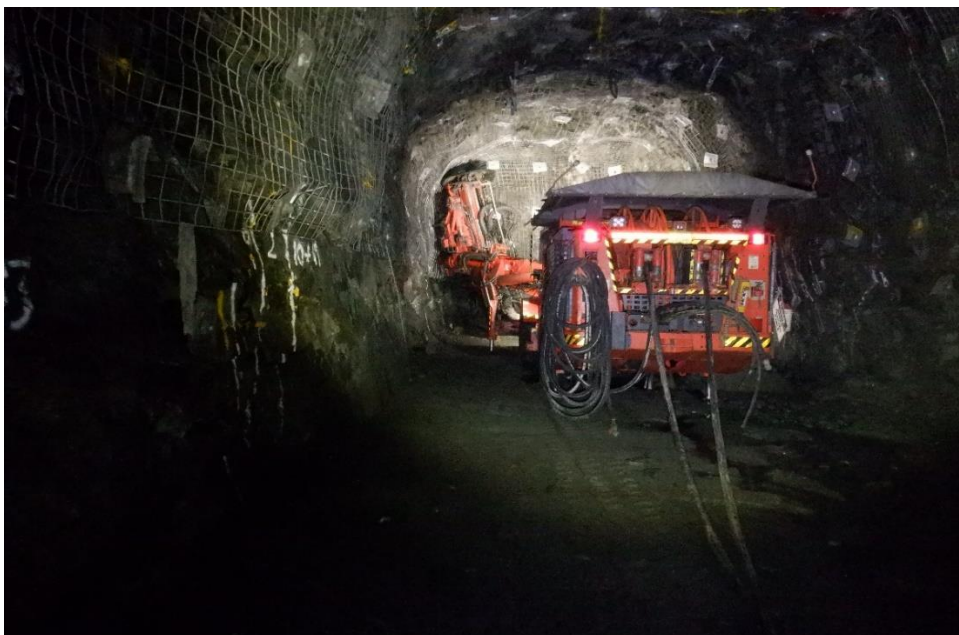
View of long drilling up holes.
