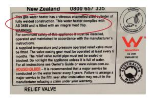
**Photo 1:** Typical data plate indicating integral heat trap on storage water heater
