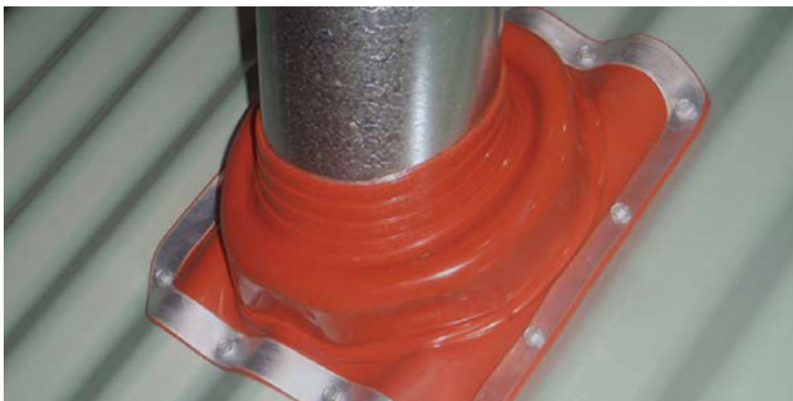
Acceptable collar flashing.
