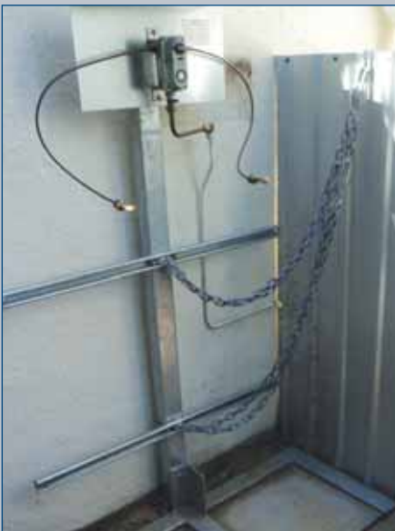
Support structure with concrete footing
