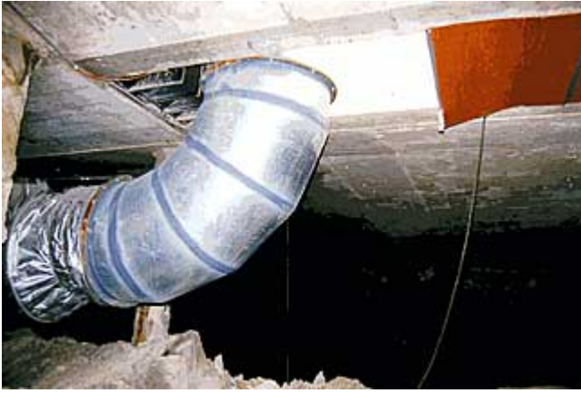
Photo 3. Intake outlet placed outside tunnel away from workers
