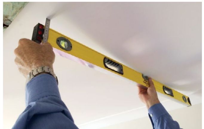
Use a spirit level to check the flatness of ceiling sheeting.
